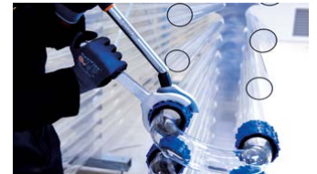
10 Next push the U-Bend over two tube ends at the same time. Afterwards tighten the blue nuts as shown, before the U-Bend is fully mounted to the system.
