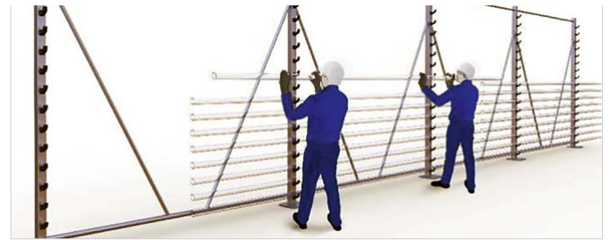
Handle glass with care: Have the tubes laid into their position by two people.
