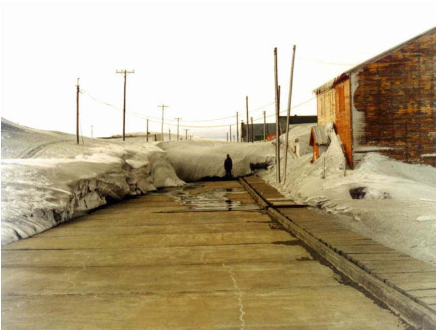
Fig. 11.9 Ice and snow from the streets of Copahue are removed by a geothermal heating system
